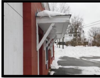
Photo Town Hall Annex 2
