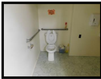
Photo Town Hall Annex 6
