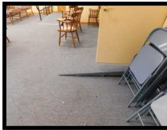
Photo Town Hall Annex 4
