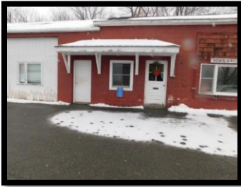
Photo Town Hall Annex 1
