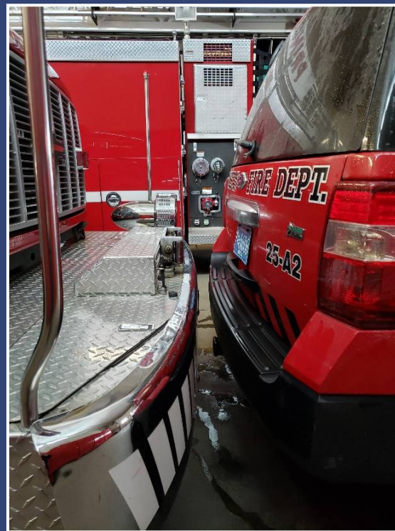
Lack of Clearance in Bays
