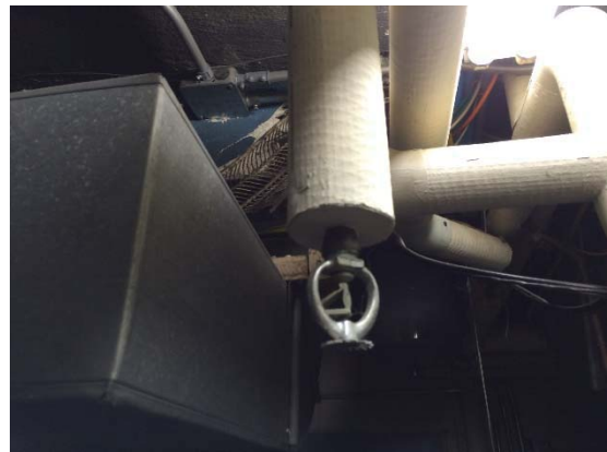
Photo 2: Sprinkler Head
