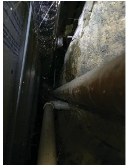
Photo 6: Piping in Cavity
