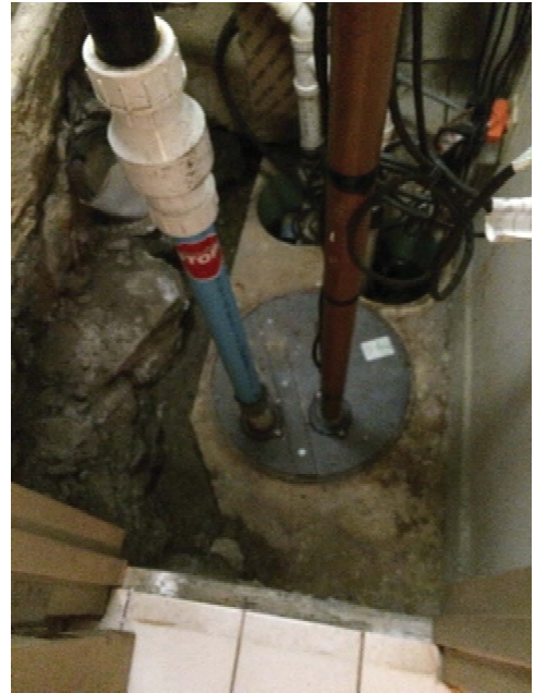
Photo 4: Sewage Ejector
