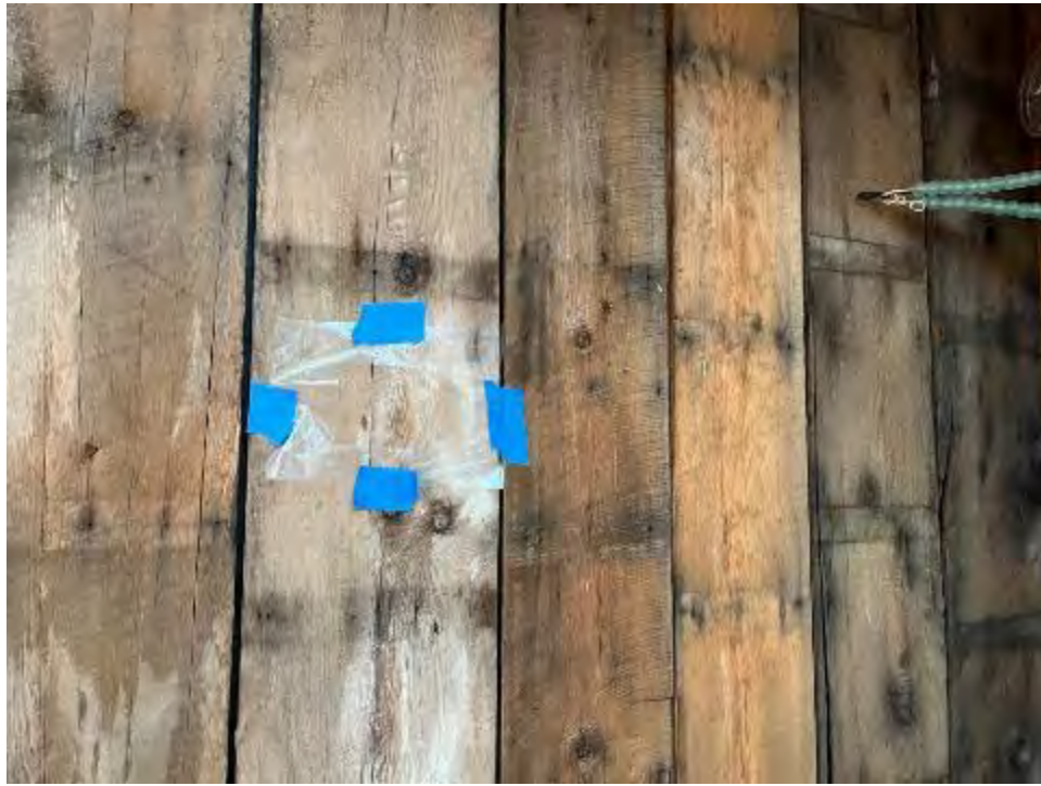
SCENE: View of wipe sample location WP-02 collected from the second floor main bedroom eastern wall.
