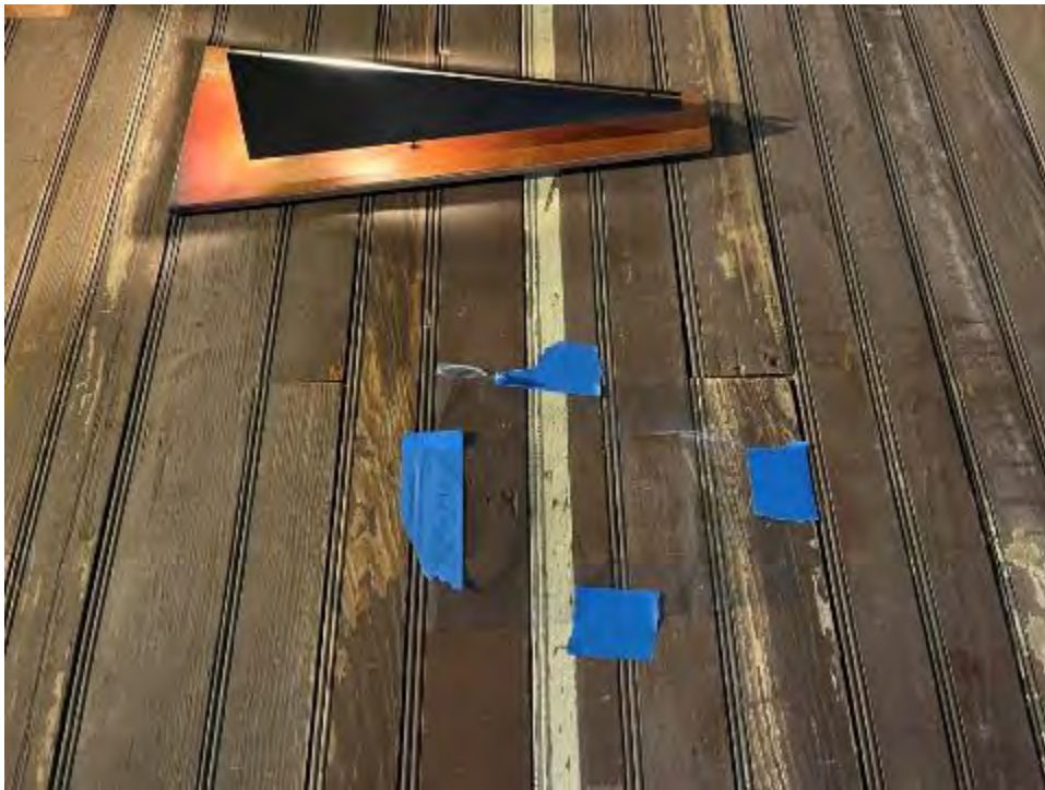
SCENE: View of wipe sample location WP-01 collected from the second floor hallway wall.
