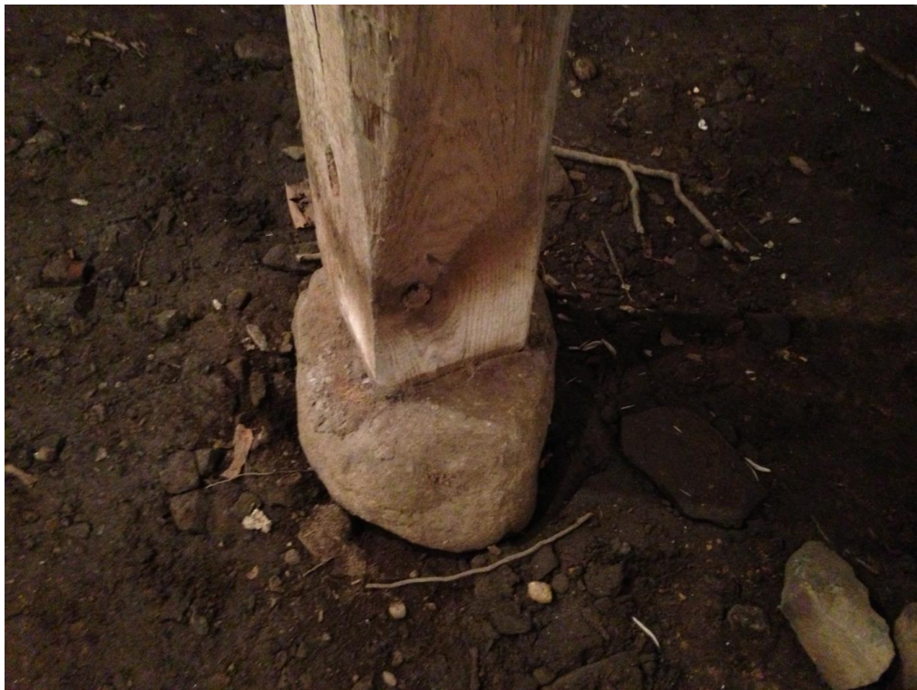
Figure 18: Rock footing for support column in the basement.
