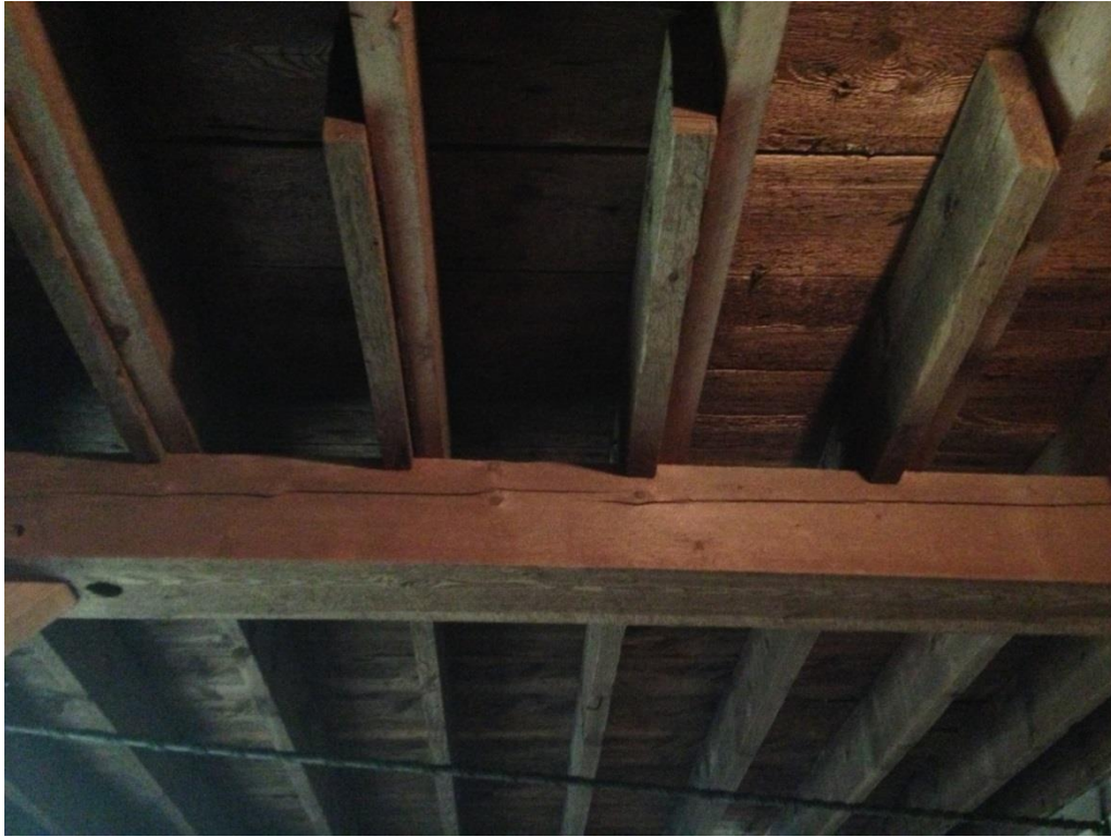
Figure 19: Framing as seen from the basement of the Addition
