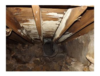
An area of damage in the Northwest corner contains compromised structural elements including apparent moisture damage to joist, girder and sill components. The damage appears to be contained to an area of four joist bays, approximately 6' in length.
