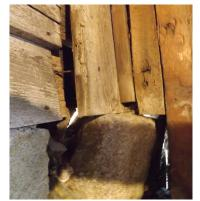
existing interior girders appear to be in sound structural condition. Many of the visible sills appear to be in sound condition as well; however, two areas were identified as being in need of repair at the Northeast and Southeast corners of the main structure, where the sills are visibly deteriorated at the corner post intersection. Additionally, portions of the sills that are not currently visible can not be evaluated until the removal of exterior sheathing takes place.
