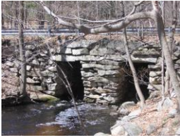
Bridge abutments & stone sluiceway on Gleason Road
