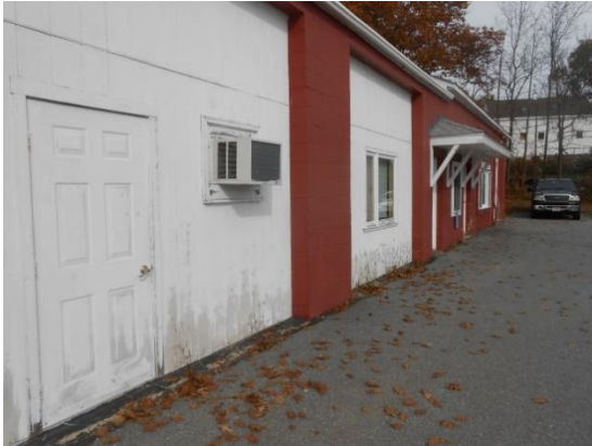
Through the Wall Air Conditioner
