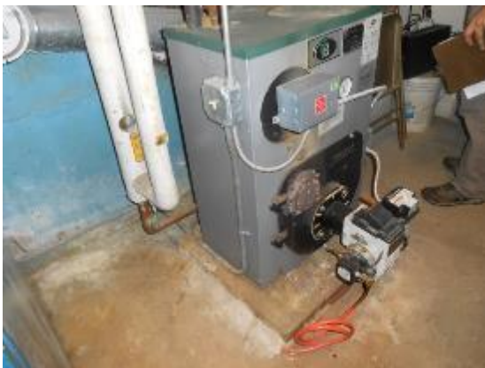
Public Safety Oil Fired Hot Water Boiler
