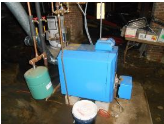
Oil Fired Hot Water Boiler
