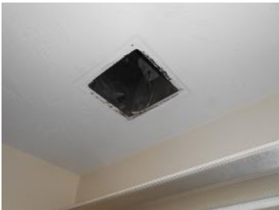
Police Station Utility Room Missing Ceiling Exhaust Fan
