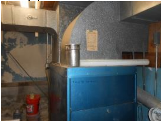
Fire Station Oil Fired Furnace w/ Distribution Ductwork
