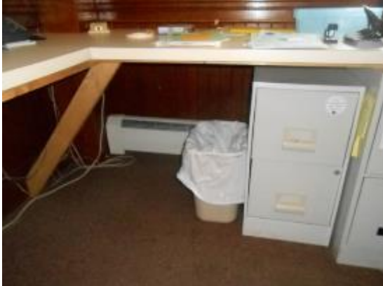
Partially Blocked Hot Water Baseboard Heat
