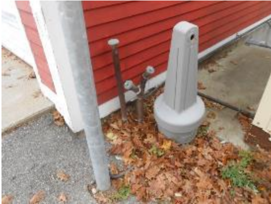
Oil Fill & Vent to be Extended
