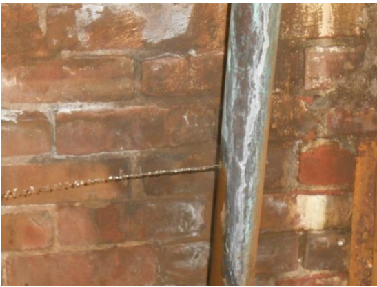
Substantial Pinhole Leak in Copper Condensate Piping
