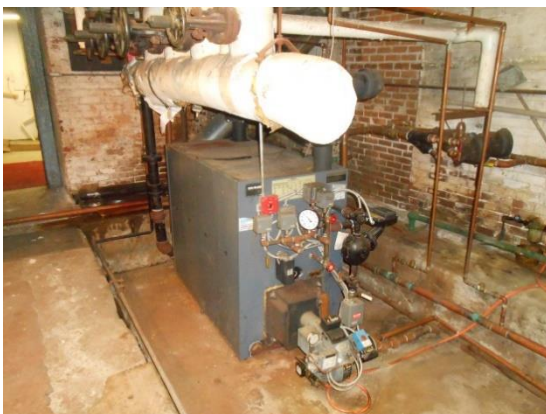
Oil Fired Steam Boiler
