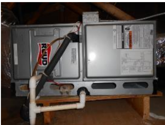
Police Station Air Conditioning Air Handler
