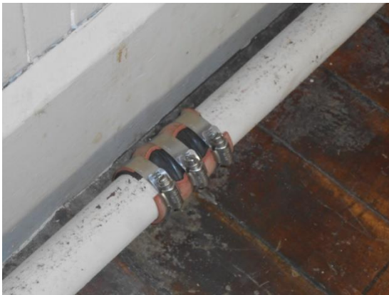
Temporary Piping Repair
